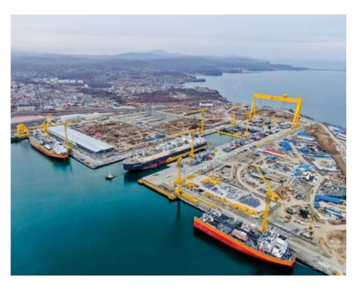
The shipyard's capabilities allow applying the most efficient method of construction – large-block construction, which is employed today by the world's leading shipyards: ships are assembled from blocks weighing **up to 3,500 tonnes**.
